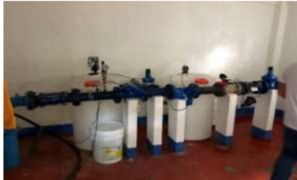
Exhibit 21.3.A.2C - New metal pipes and chlorinators.
